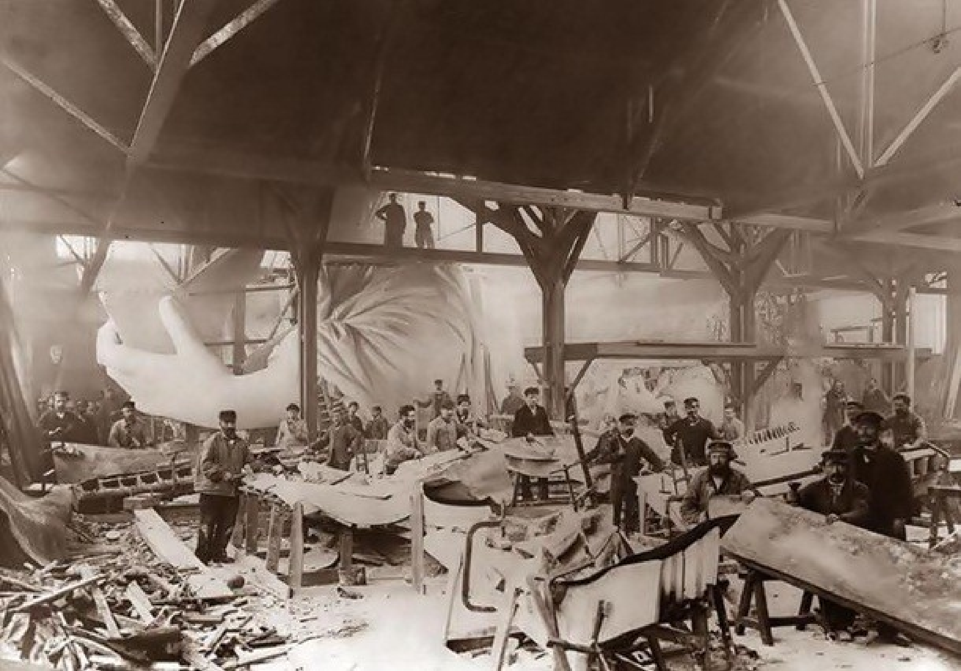
The construction of the Statue of Liberty in 1884
