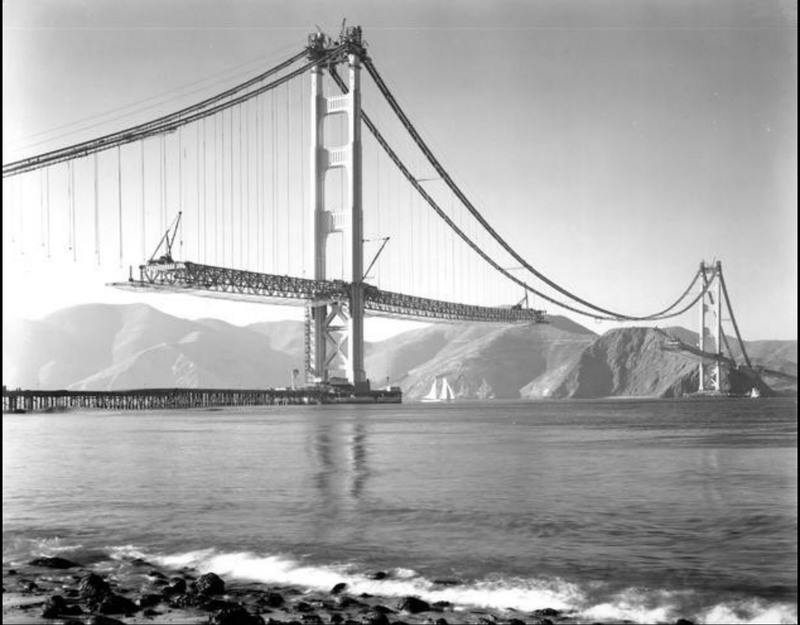
Golden Gate Bridge construction 1937
